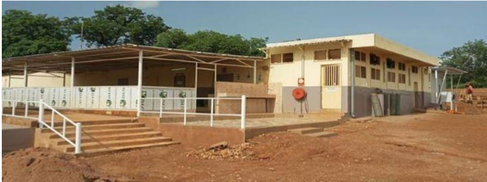
Mess Facility Upgrade
