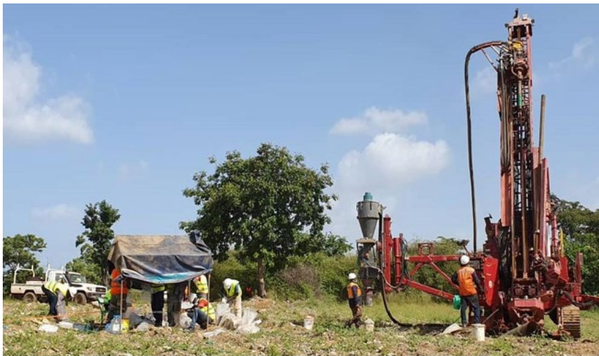
AMS Control Drill Rig
