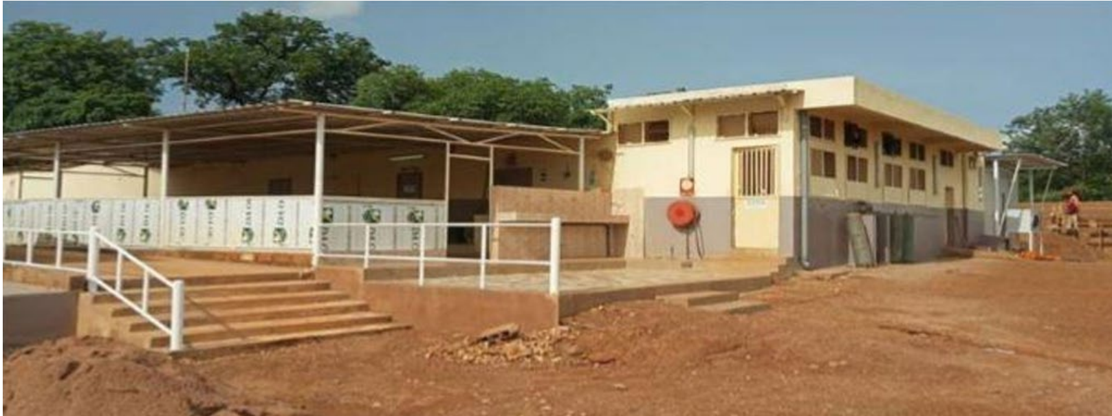
Mess Facility Upgrade
