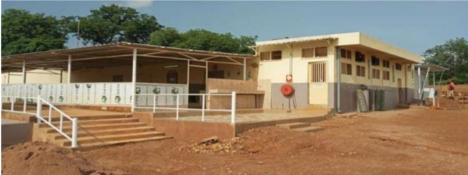
Mess Facility Upgrade
